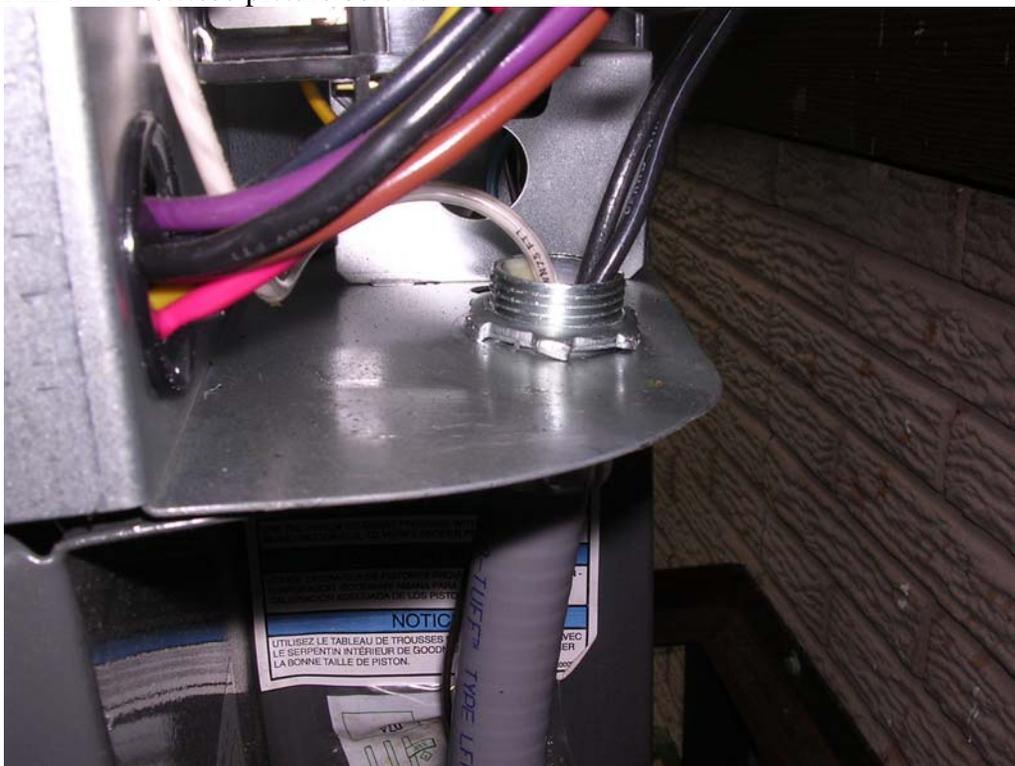
4. Make sure ALL your connections are TIGHT!...the BLACK wires connect to the 2 available screws...make you sure you are using the correct gauge wire....I am using 10 for example... you also need to connect to the thermostat...you can use wire nuts for that (not shown) see picture below...
