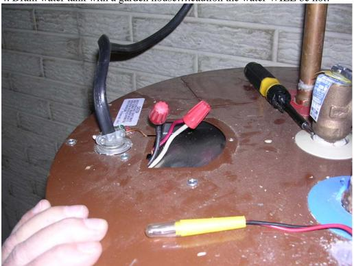
5. After you have confirmed that power and water are OFF....note the color wires and wire nuts.....a tip....green will be ground....ALWAYS test wires for safety! Again 220 will KILL you!
